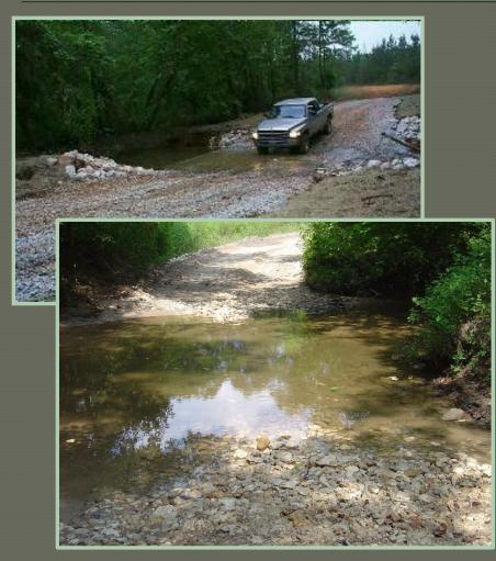
A permanent crossing for low flow streams with low banks and a firm stream bed suitable for driving across
