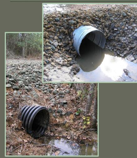
A conduit or pipe through which surface water can flow under roads that cross streams
