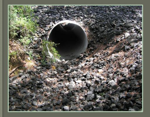
Rip-rap or aggregate placed at the outlet of a culvert or water-control device to reduce erosion
