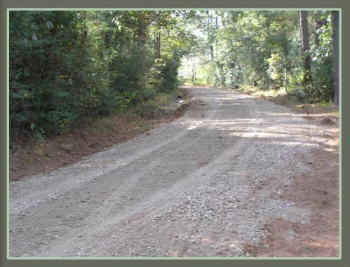
Aggregate placed on road ways to reduce the impact of rain or surface runoff
